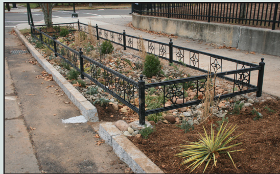
Curb Inlet Planters
